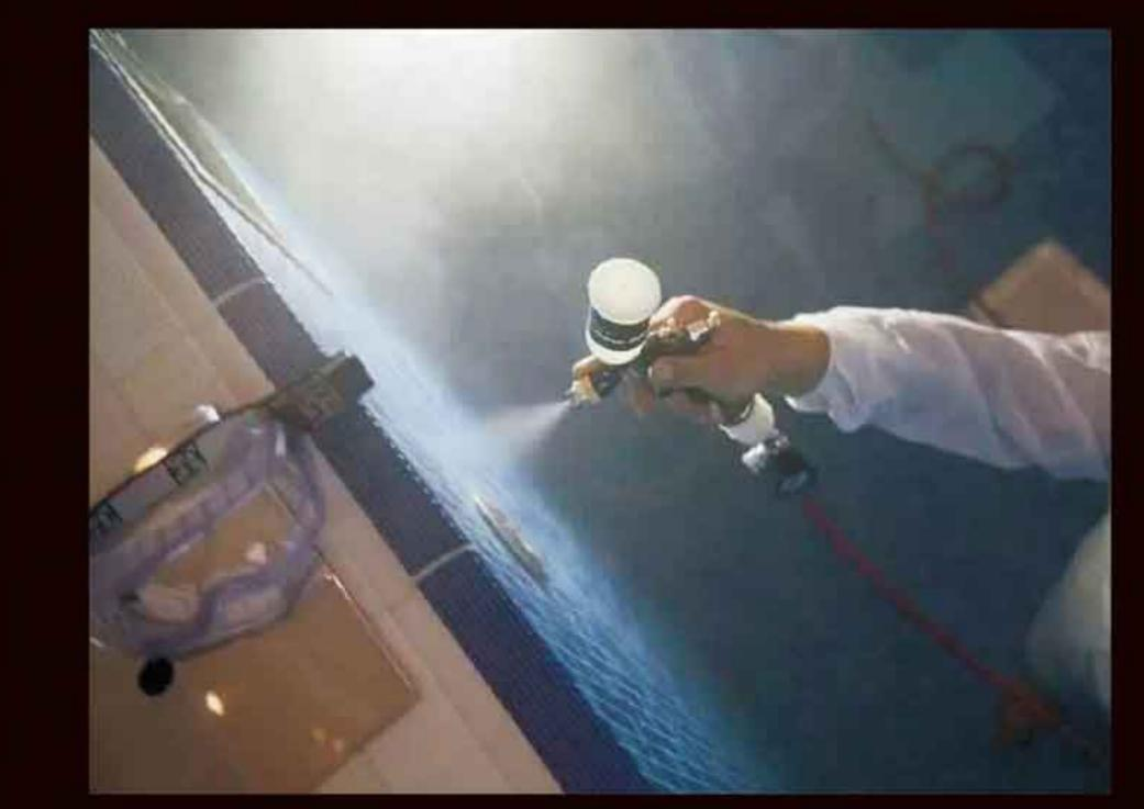
Spraying: This will result in an even thickness and a smooth surface. A dust-free environment is recommended during application.
